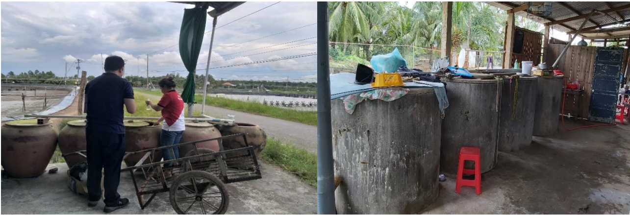
Figure 3-4: Setups of Rainwater Harvesting System at Survey Sites.
