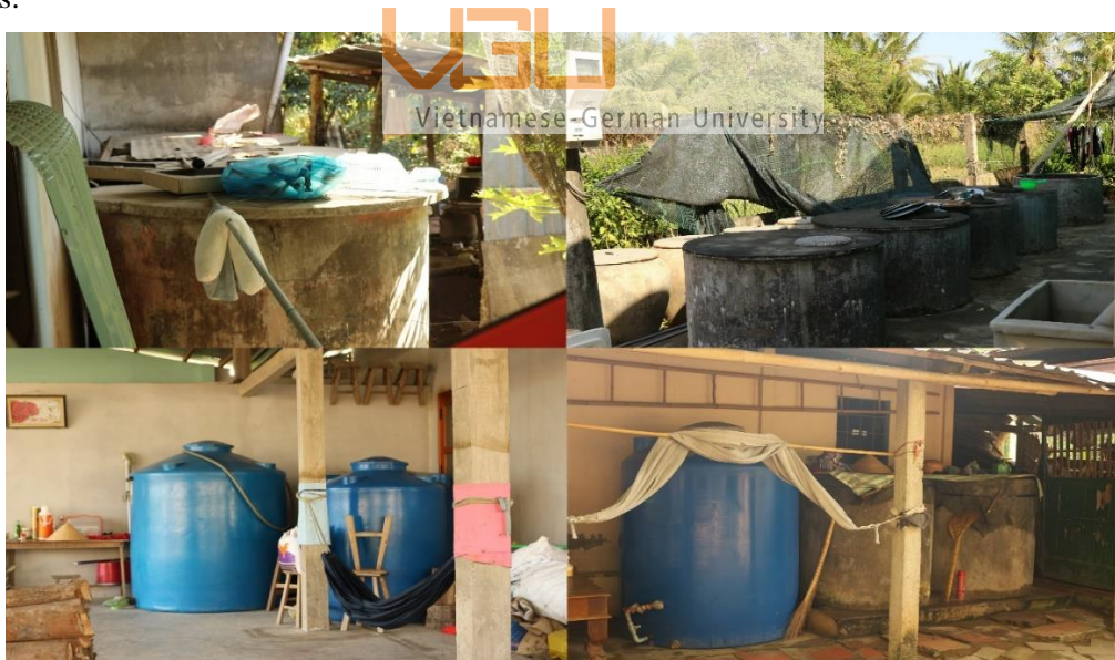
Figure 1-5: Common Rainwater Storage Used in the VMD
