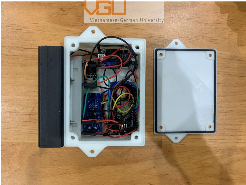
Figure 45 NodeMCU enclosure fully installed
