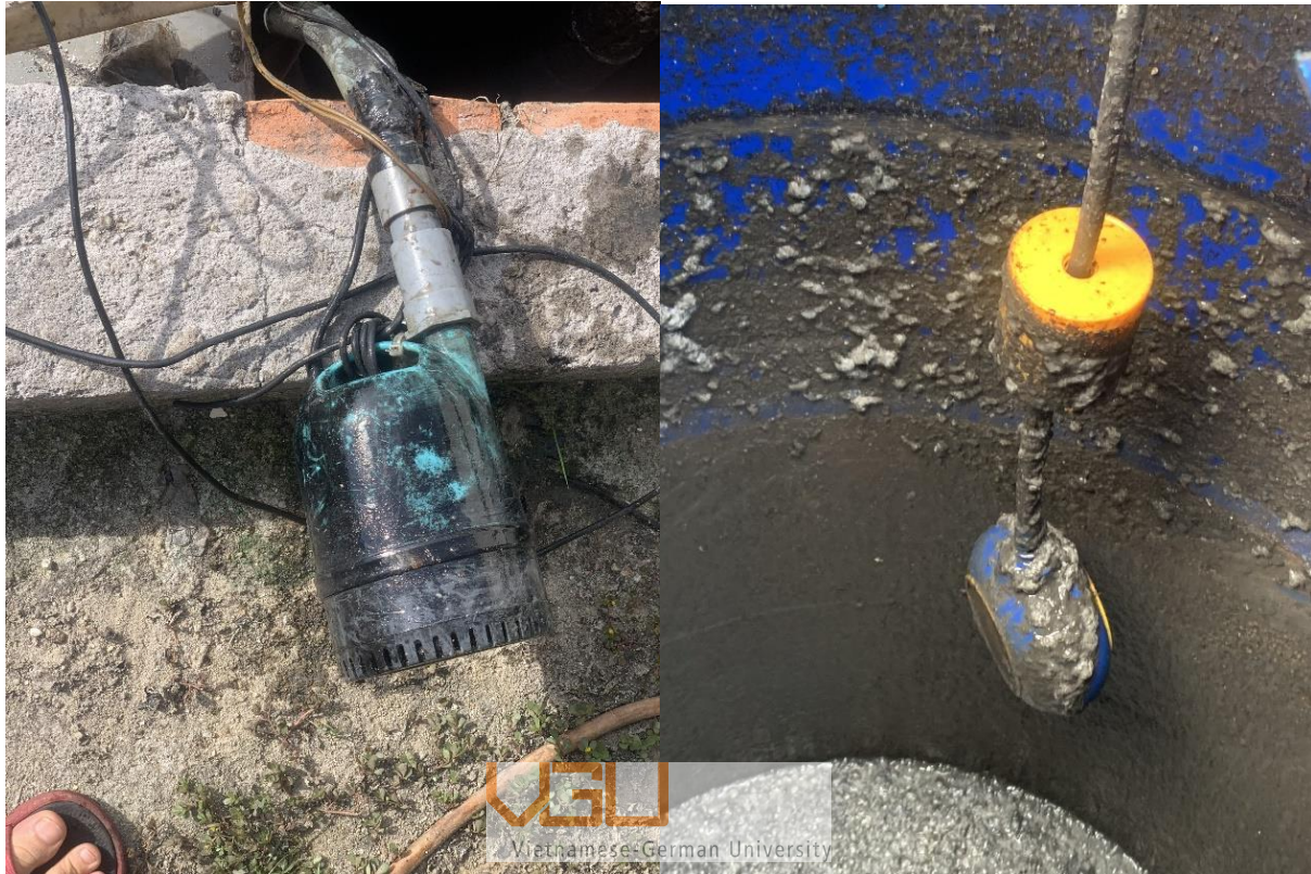
Figure 28: Submersible pump with float switch
