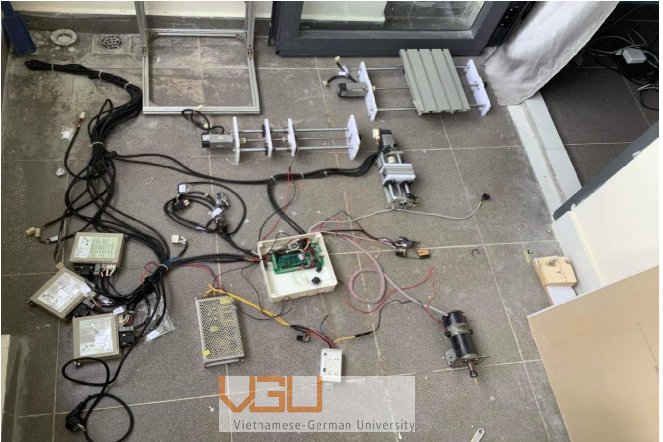
Figure 4.1: The wiring of the whole machine
